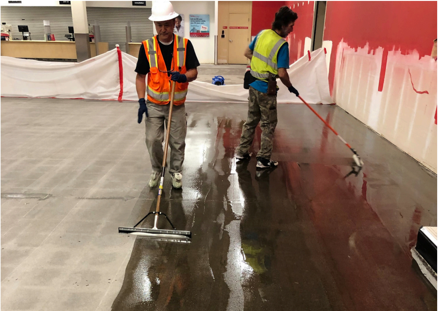
INSTALLATION OF AVM GAS-LOCK® 420
